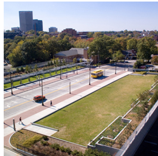
5th Street Bridge After Improvements (Source: Georgia Institute of Technology)
